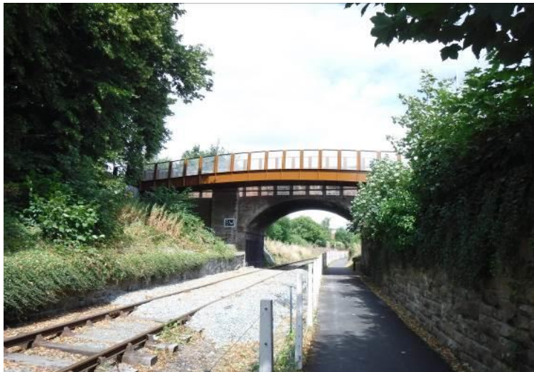
Lys Lane Footbridge – Bridge Replacement
